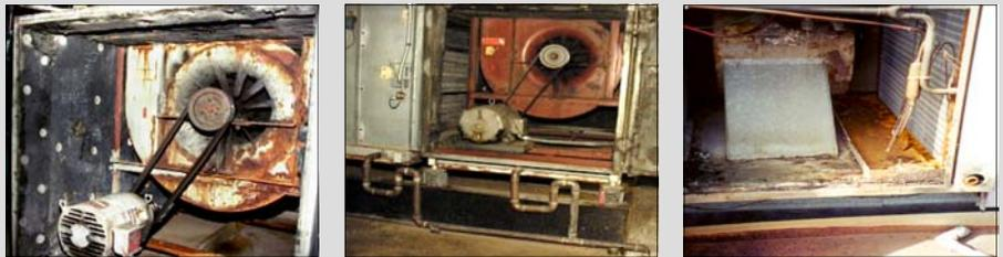
FIGURE 2 Air Handlers - Contaminated and Damaged
