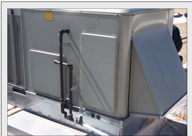
Figure 4. Typical installation of a CostGard™ Condensate Drain System
