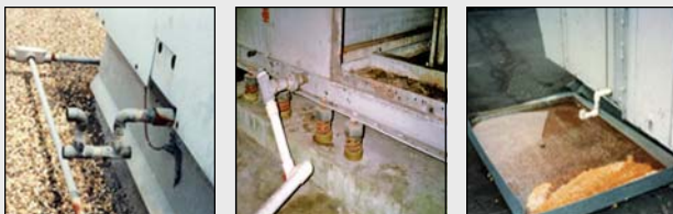
Figure 1. Typical trapped systems that meet industry codes
