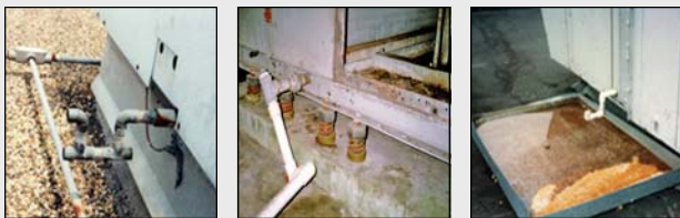
Figure 1. Typical trapped systems that meet industry codes
