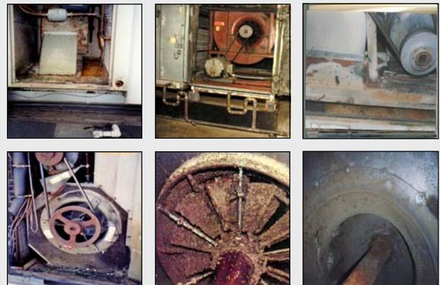
**Figure 2.** Damaged and health threatening air handlers caused by failed drain systems
