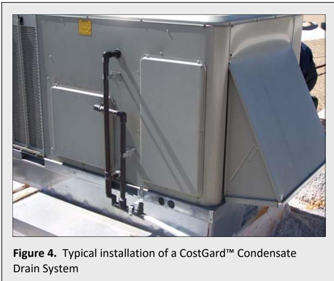
**Figure 4.** Typical installation of a CostGard™ Condensate Drain System
