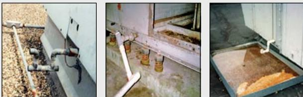
**Figure 1.** Typical trapped systems that meet industry codes
